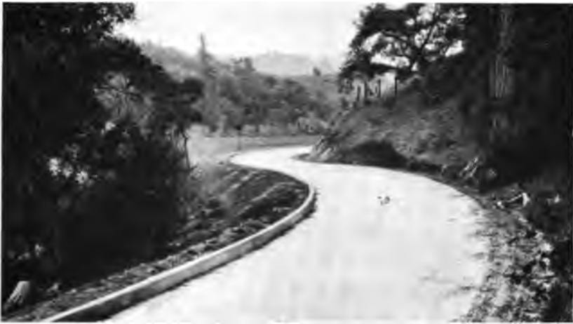
Concrete curb, in addition to preventing roadside wash, supplies a measure of safety.
